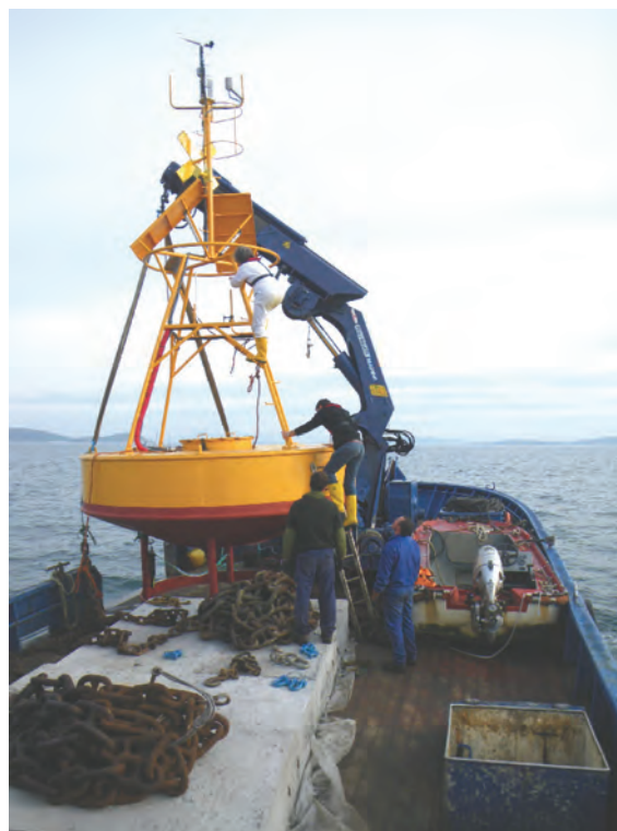
Fig. 3. Mooring maneuver of one of the buoys.
