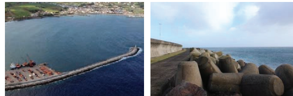
Fig. 1. Left: aerial view of Praia da Vitória Port, with the South Breakwater and Quay 12 in the foreground. Right: detail of South Breakwater crest.
